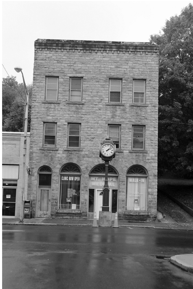
6. Mount Hope Bank Building facade, looking northwest with new noncontributing clock shown in the foreground
