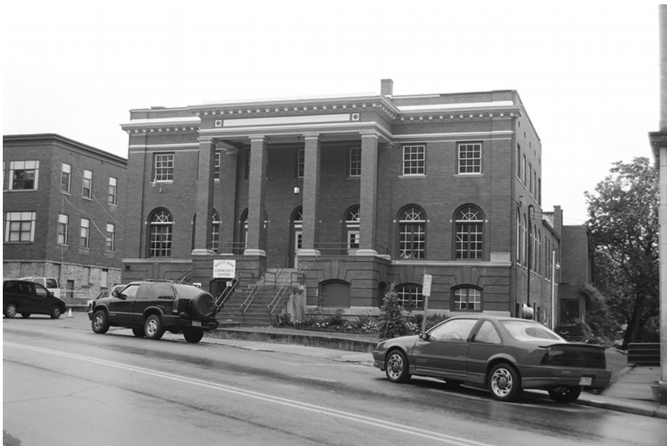
10. Mount Hope YMCA/Community Center, looking southeast, with one of the vacant school buildings shown at the left.
