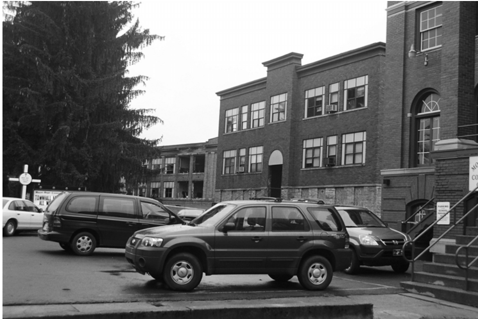
11. Vacant school buildings, Main Street, looking east, with the corner of the YMCA/Community Center visible at the right.
