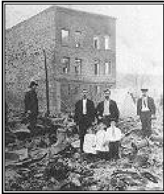
Fig. 2 This view of the Bank of Mount Hope (Resource No. 34) shows it to be among the few properties left standing after the 1910 fire. [from Peters and Carden]
