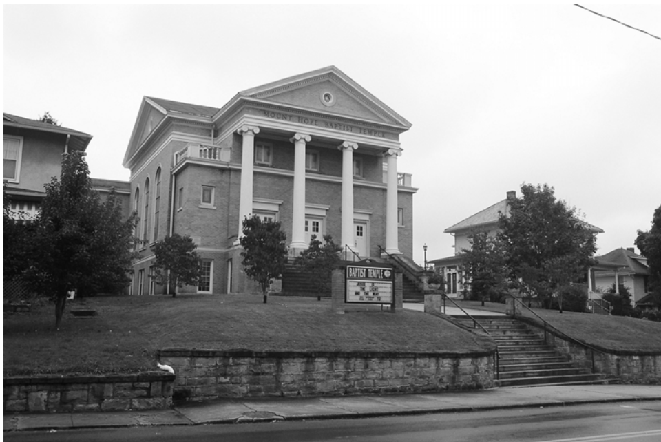
20. Mount Hope Baptist Temple, facade, showing Main Street elevation and substantial stone retaining wall along the front perimeter of the lot.
