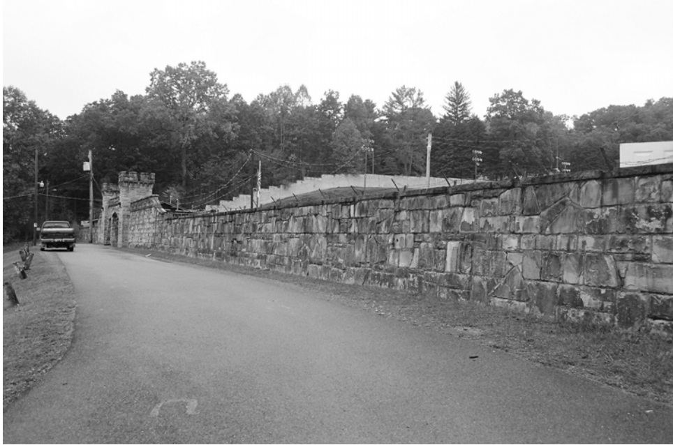
13. Mount Hope Municipal Stadium, exterior wall on south perimeter, showing overall character of the wall, and crenellated entry portal at left.
