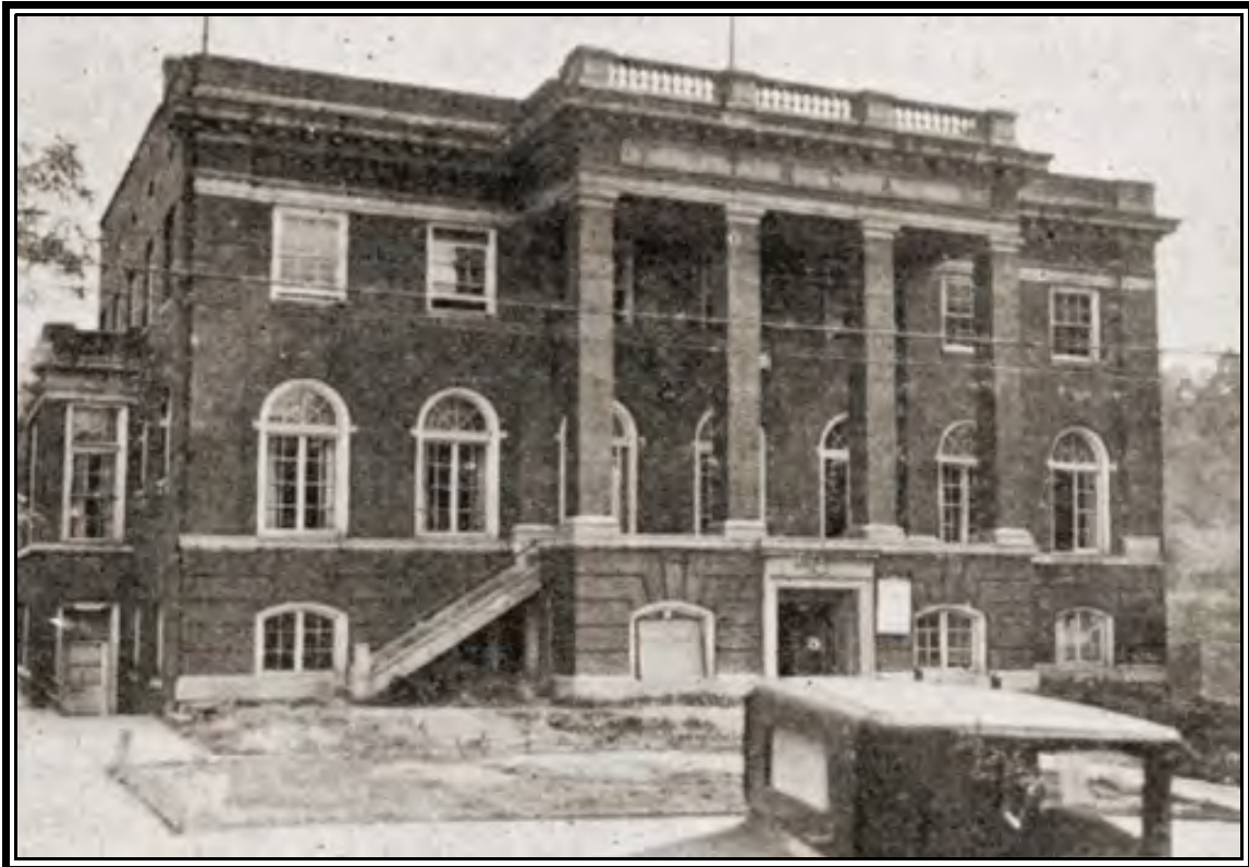
Fig. 11 The YMCA, now known as the Community Center (Resource No. 1), shortly after its 1921 construction. [from Peters and Carden]
