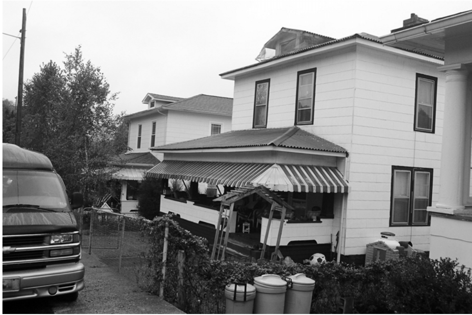
17. Streetscape, Madison Street, showing repetitive American Foursquares at 304 and 306 Madison, looking northeast.
